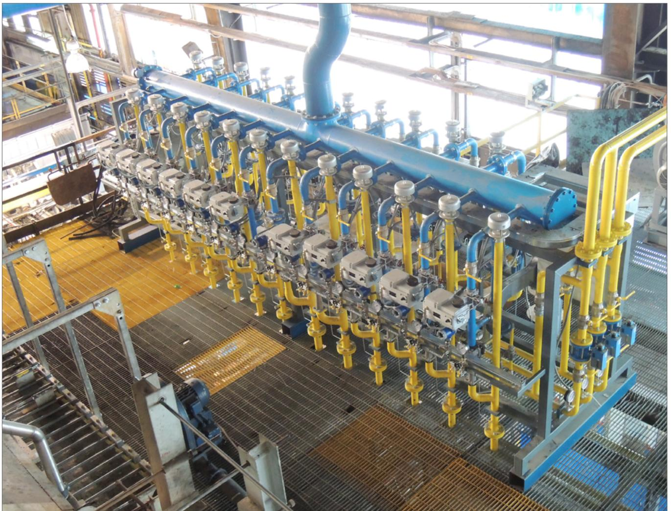
The forehearth & distributor combustion skid designed by **Glass Service** are compact and easy to install.
