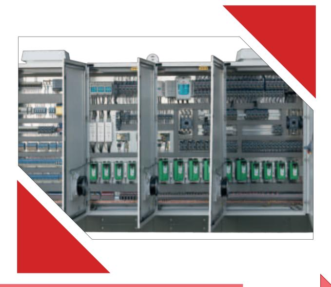
The simplest control architecture proposed as standard by Glass Service includes a system based on a PLC/DCS with one CPU + various I/O boards and an HMI touch screen user interface.
