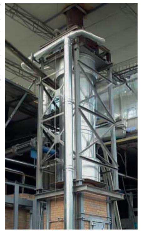
Typical configuration with double stage recuperator
