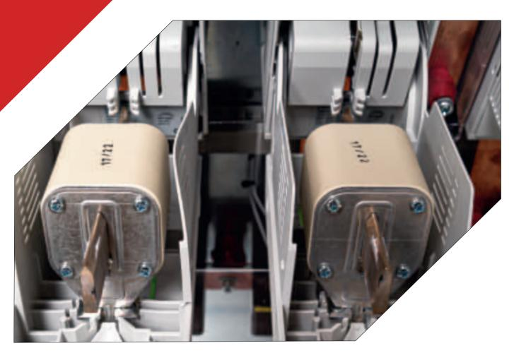
Output fuse open, one for each electrode
