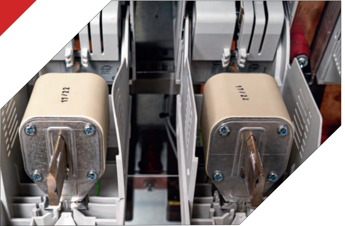
Output fuse open, one for each electrode
