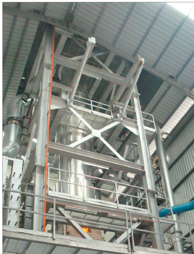
Typical installation of a single stage recuperator over furnace stack
