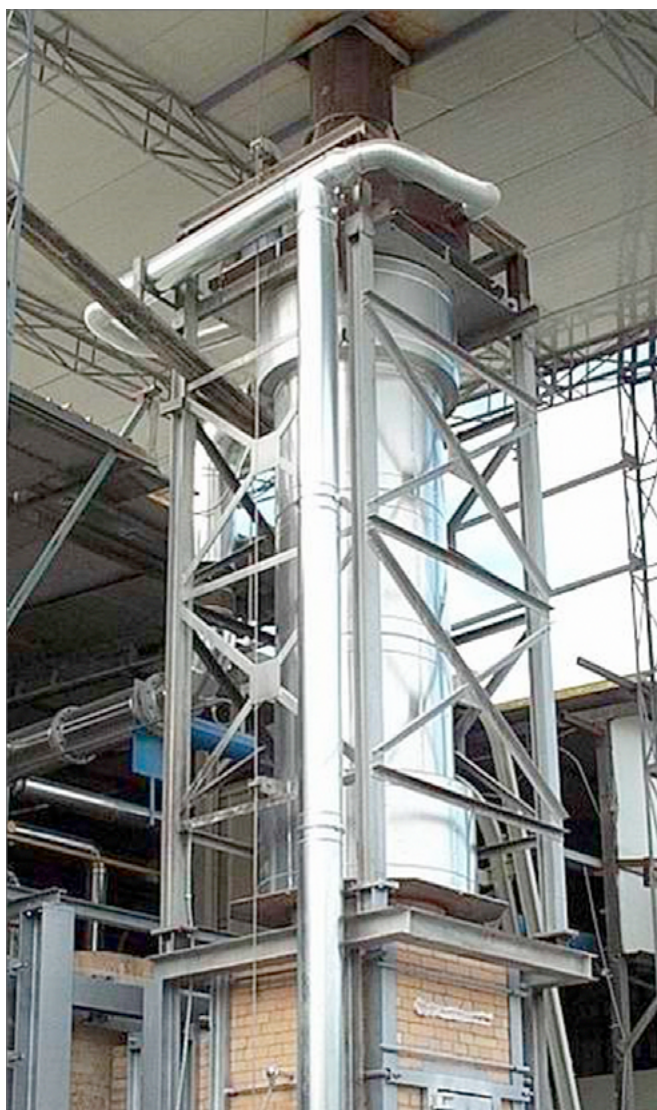
Typical installation of a single stage recuperator over furnace stack
